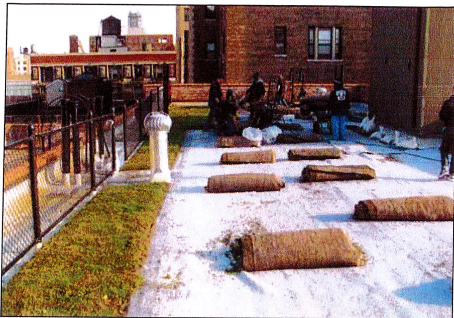
Pre-vegetated green roof mats roll out like sod.
