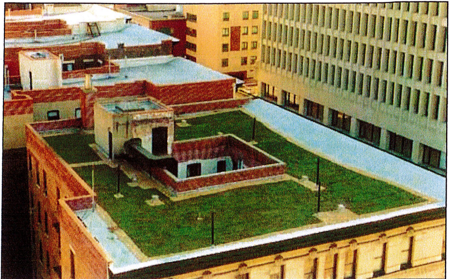
Columbia's seven green roofs reduce stormwater runoff.
