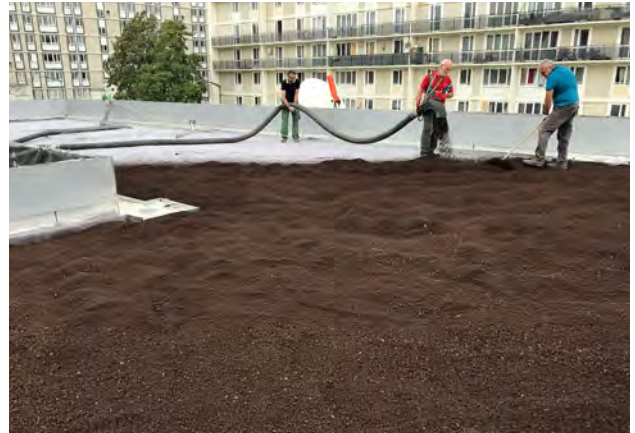
Substrate installation blower truck for a nursery roof (France) Credit: Dynergis
