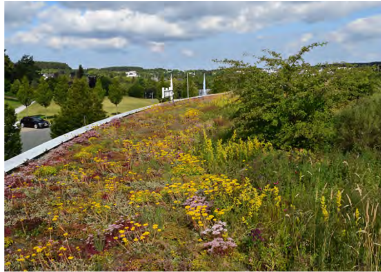
Semi-intensive green roof, Germany
