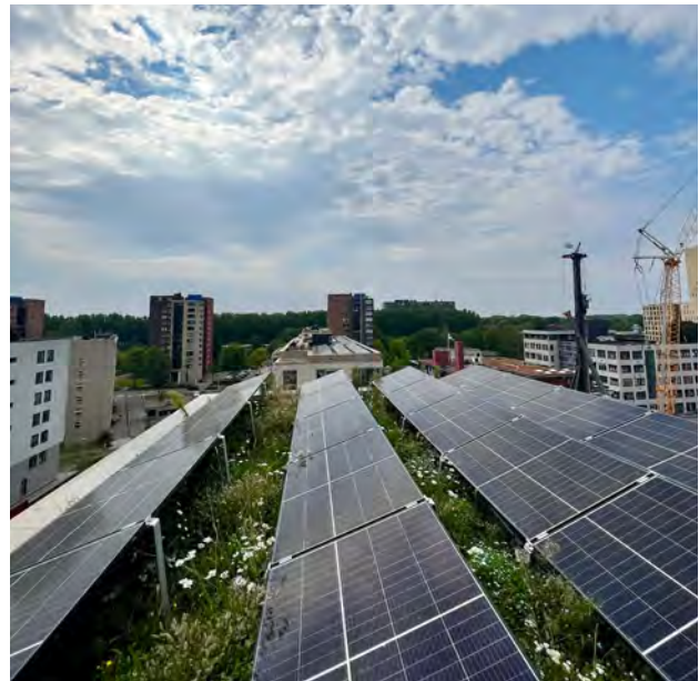
Oblique panels on a solar green roof
