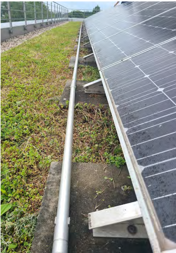
Pavers used to ballast solar panels are placed on the green roof along with electrical conduit. Credit: Steven Peck
