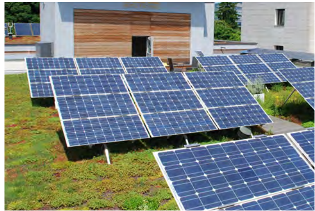
Solar green roof, Germany Credit: BuGG
