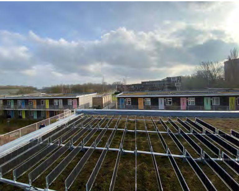
Vertical bifacial solar green roof on a multi-unit apartment building in Amstelveen, Netherlands Credit: Over Easy Solar
