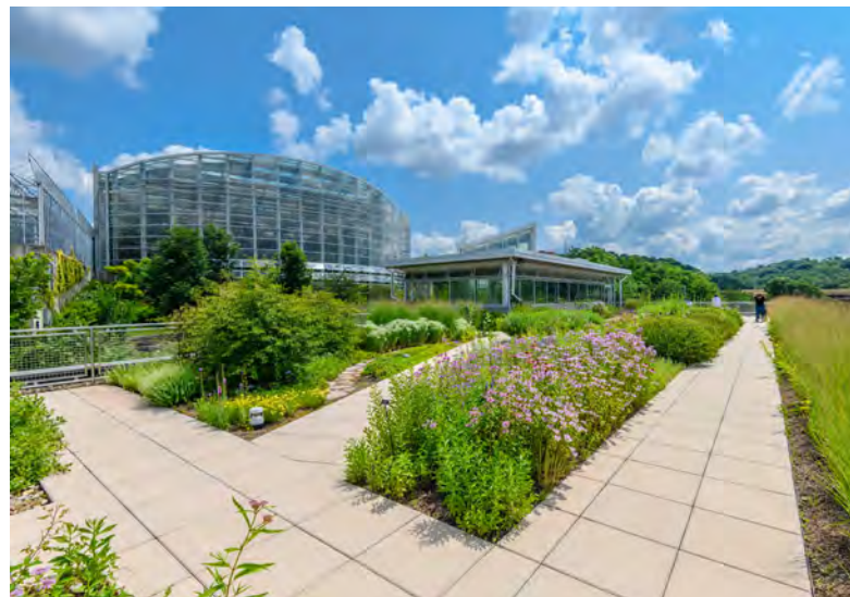
Phipps Center for Sustainable Landscapes - Green Roofs for Healthy Cities Awards of Excellence Winner 2020 Intensive green roof installed installed as part of a larger ecological system at the Phipps Conservatory in Pittsburgh PA.
