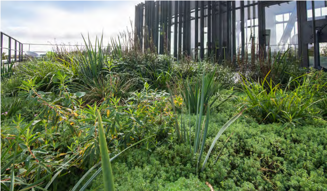
The green roof of this laboratory has been designed to manage rainwater in order to promote evapotranspiration by plants. Credit: Sopranature
