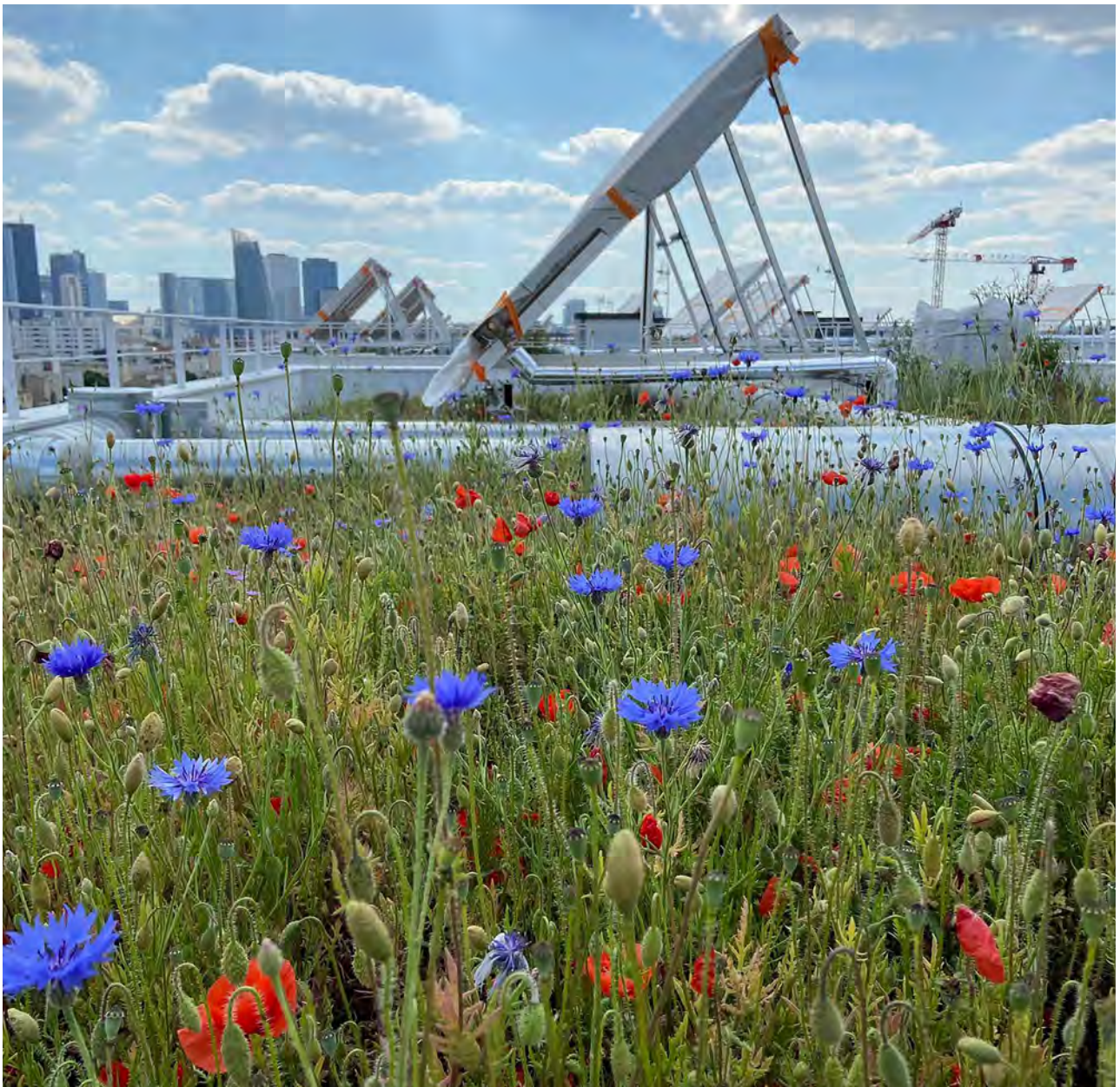
Thermal solar green roof installation about to be finalized (Village Delage, Courbevoie, France)
