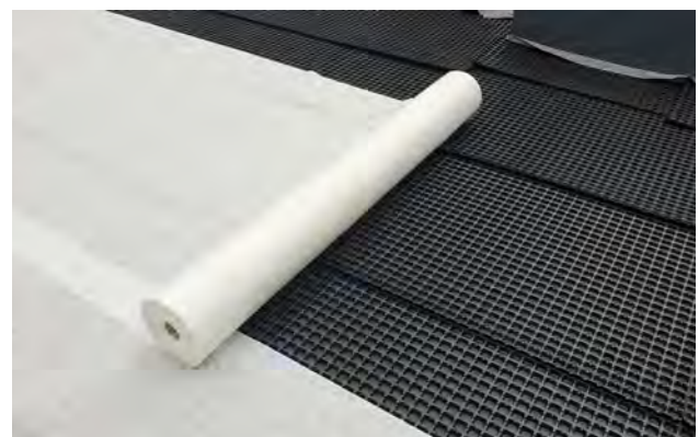
Filter fabric being unrolled over the drainage layer Credit: Christian Oberbichler, Dachgrün GmbH
