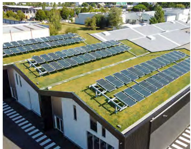
Solar green roof integrated project in France Credit: Vegetek
