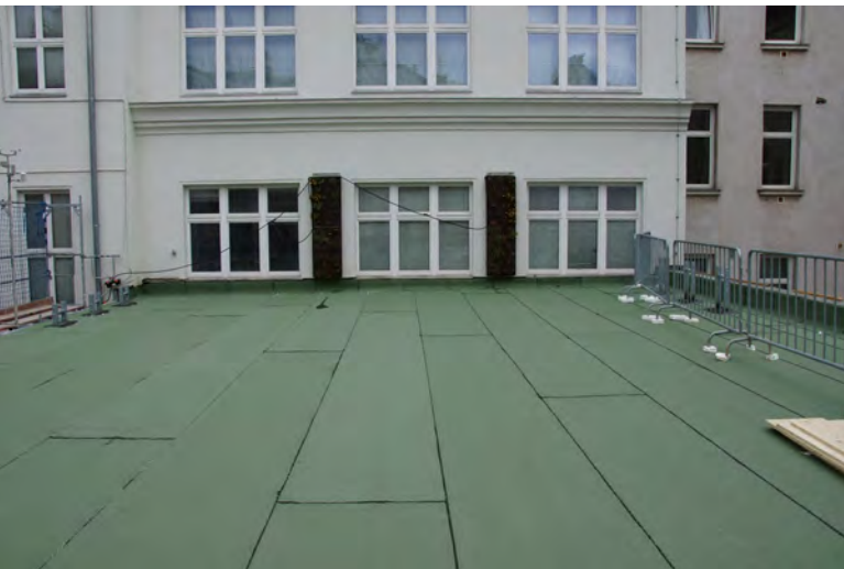
Waterproofing membrane being installed
