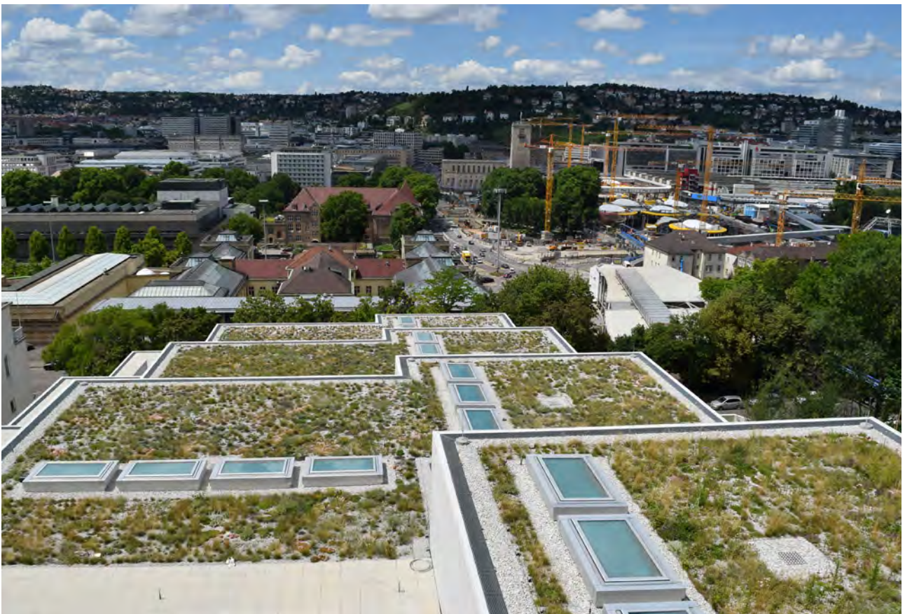
Extensive green roof in the city center of Stuttgart Credit: BuGG
