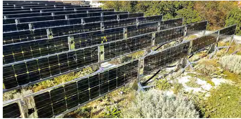
Vertical Bifacial System Credit: ZHAW, Dreisiebner
