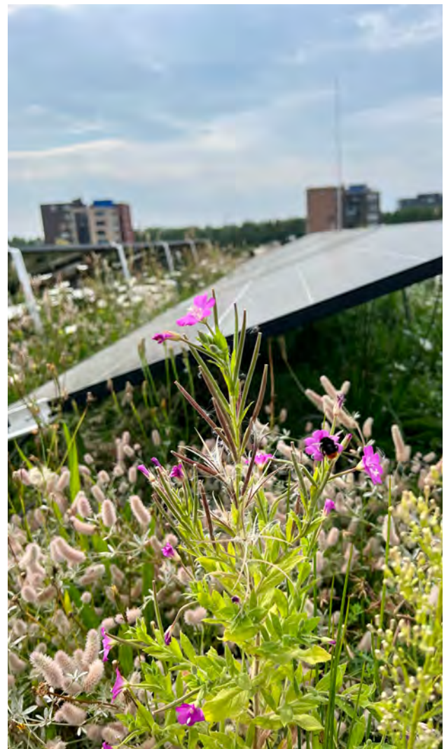
Solar Green Roof integrated project Credit: Permavoid
