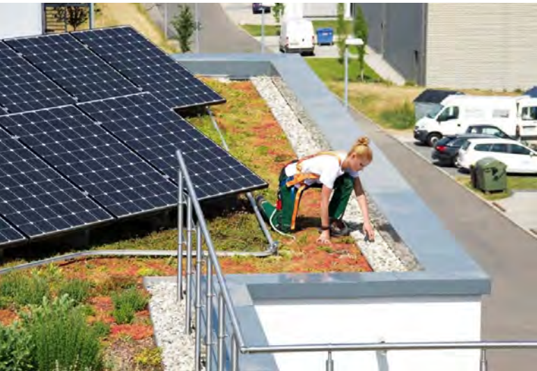
Maintenance of a Solar green roof Credit: ZinCo AG
