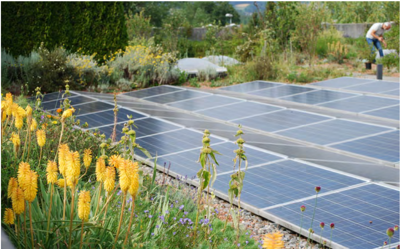
In some cases, the roof design as well supports a division of technologies (Switzerland)
